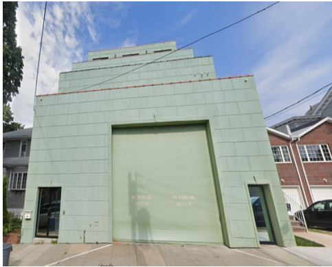
14-07 113th Street 14-07 113th Street College Point, NY 11356
