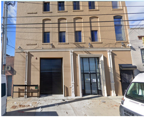
15-32 127th Street 15-32 127th Street College Point, NY 11356
