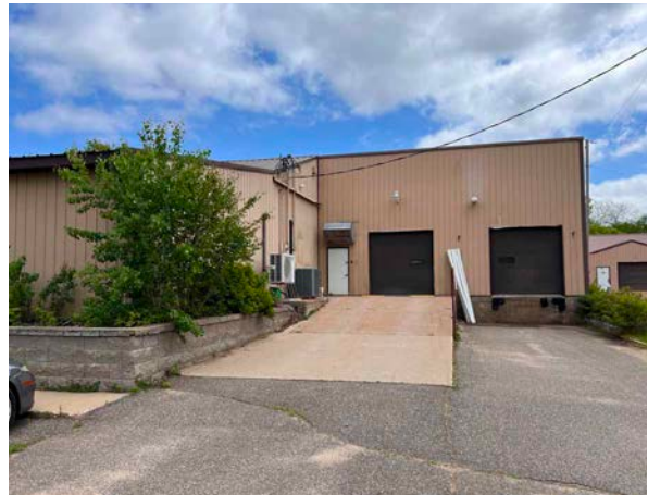
Building #1 / Suite #1 - Drive-In Door & Loading Dock
