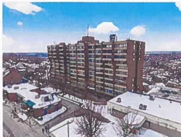
Front of Structure
