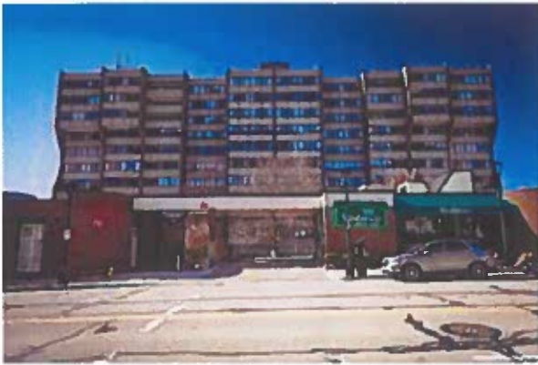
Front of Structure - Welcome to the Washington Square Condominium and office building in the Uptown business district of Mt Lebanon. Adjacent to the parking garage and public parking lot, this central location is highly visible and easy to navigate clients accessibility.
