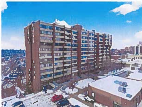
Front of Structure
