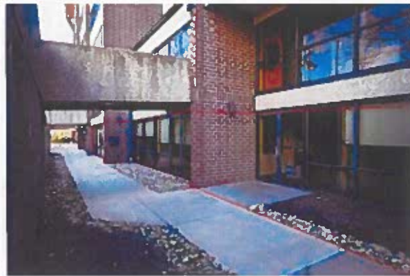
Front of Structure
