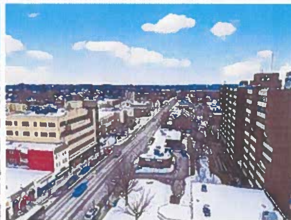
Aerial View - Southern view.
