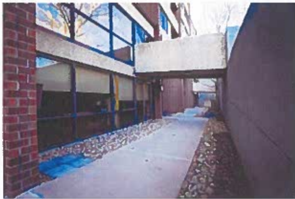
Front of Structure - Walkway on lower right portion of the building with 2 entrances from the front sidewalk.
