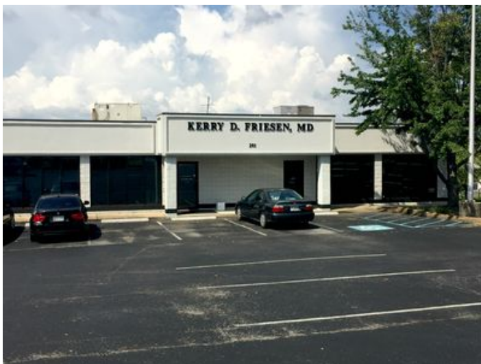
Rear View of Bldg
