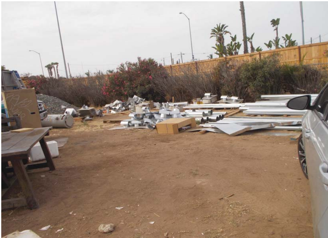
2) View of typical construction equipment on vacant portion of Site.
