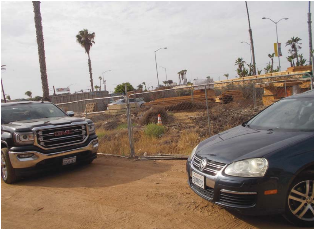
1) View of typical debris piles on vacant portion of Site.
