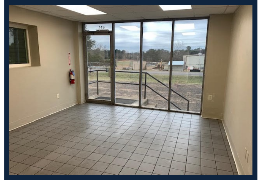
Front Entry Office or Display Area
