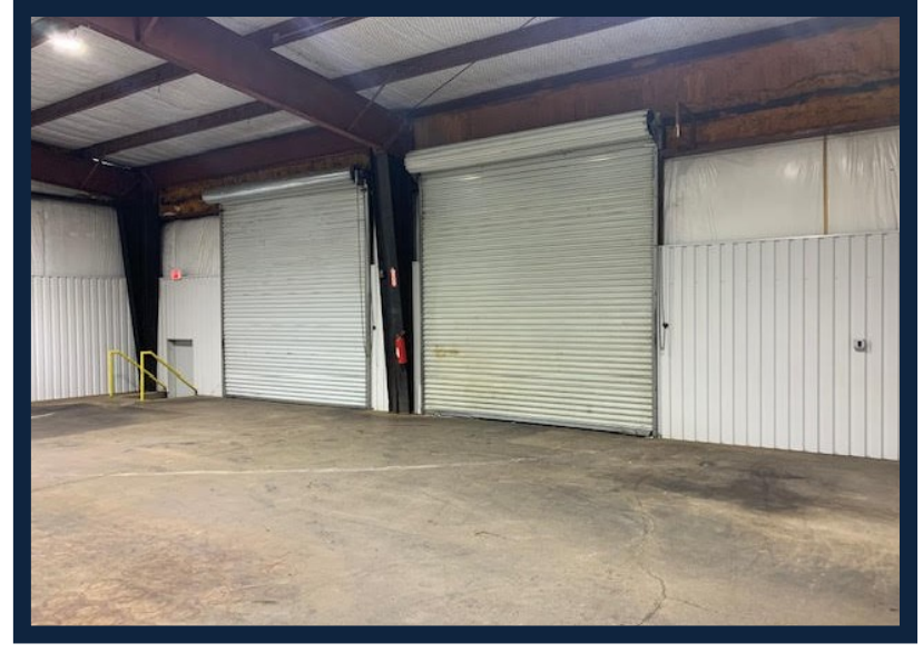
South Side Two Dock Doors
