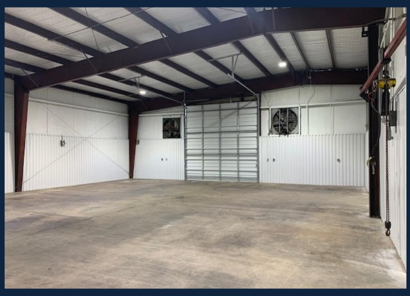
Warehouse Area with East Side Ground Level OH Door
