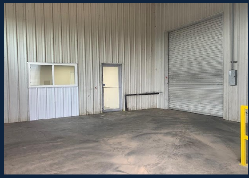
Covered Dock Space with Ramp Access
