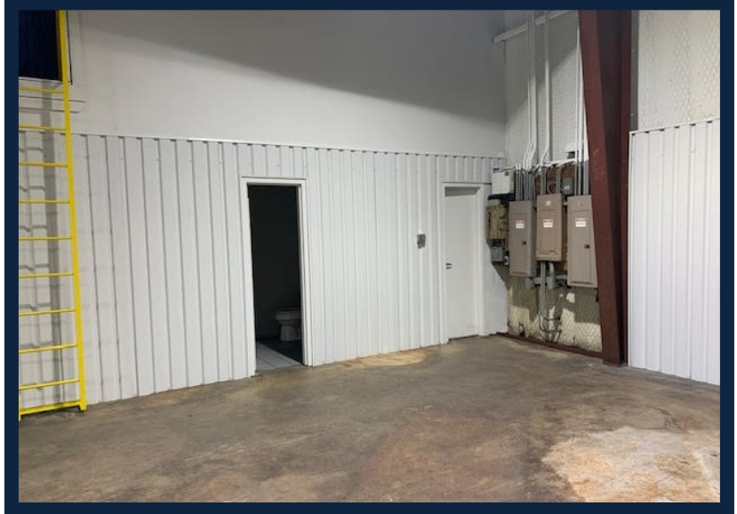
Two Restrooms in Shop
