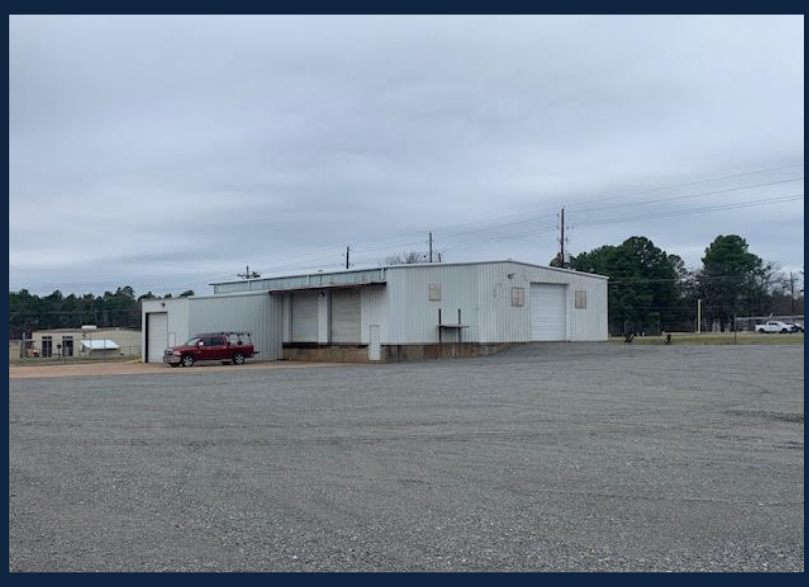
Photo From SE Corner Looking Back on Office Warehouse
