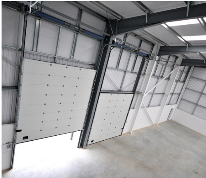
Previous Chancerygate units similar to unit 6.
