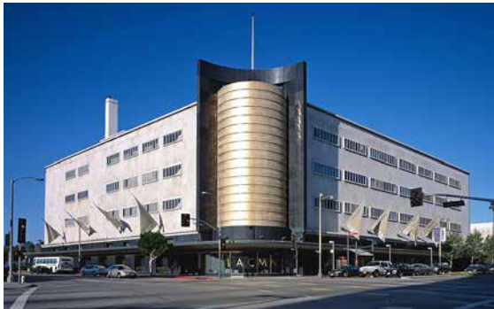
The 1939 Streamline Moderne May Co. Bldg
