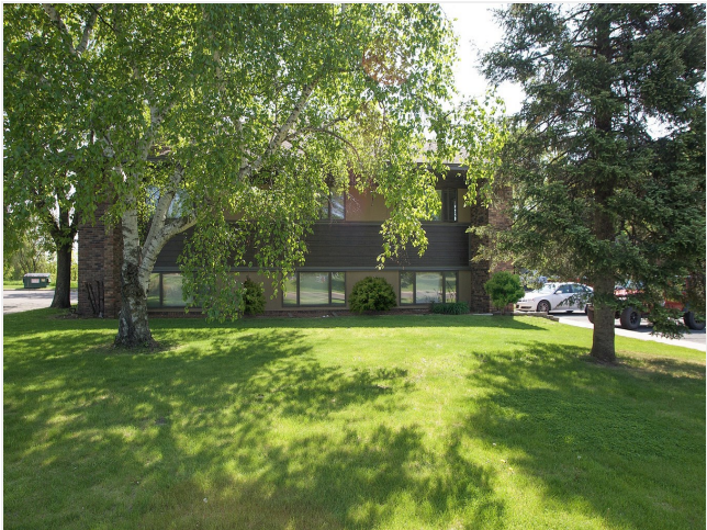
West side of the office building
