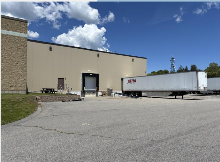
Two (2) Dedicated Tailboard Docks
