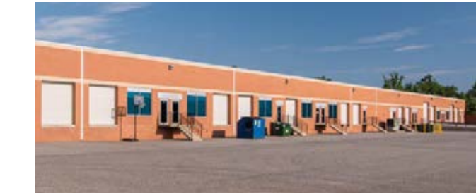
Flex/R&D dock and drive-in loading
