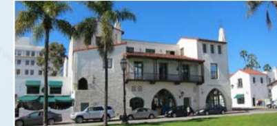
740 State St., 3rd Floor ±4,309 SF Retail Building
