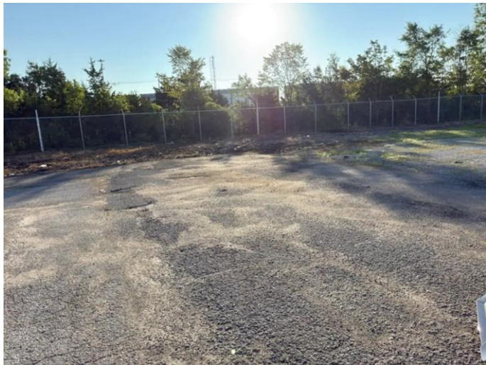
Perimeter fence line along the site
