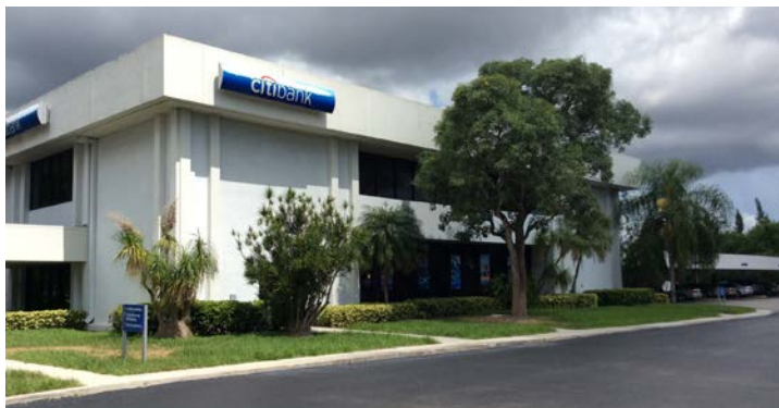
View of east side of building
