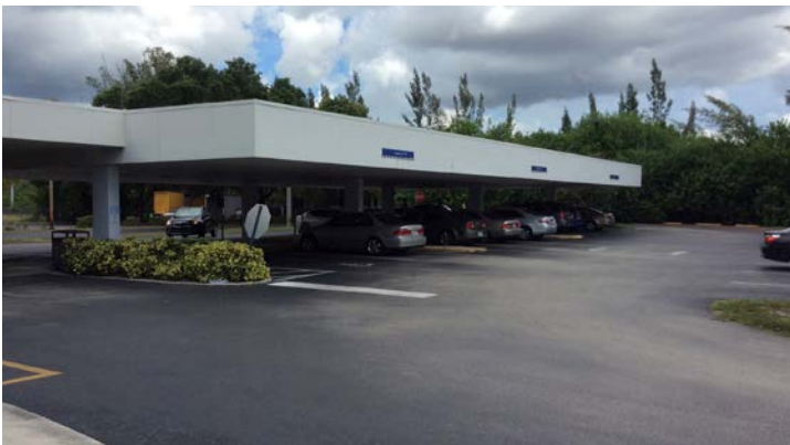
View of covered parking
