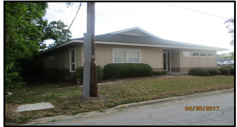
View Of The Northern(Front) And Eastern Elevations
