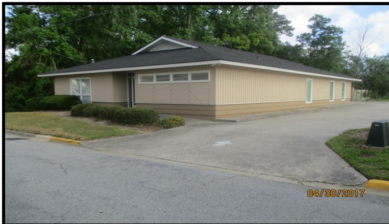
View Of The Northern (Front) And Western Elevations
