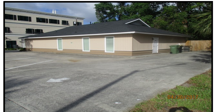
View Of The Southern (Rear) And Eastern Elevations
