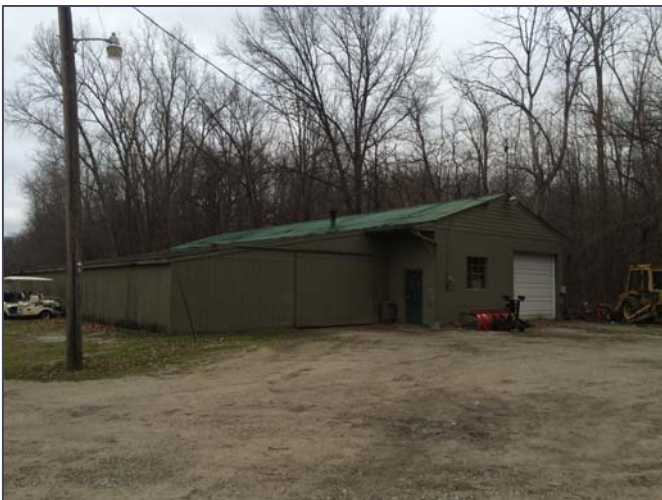
4,500 square foot maintenance building
