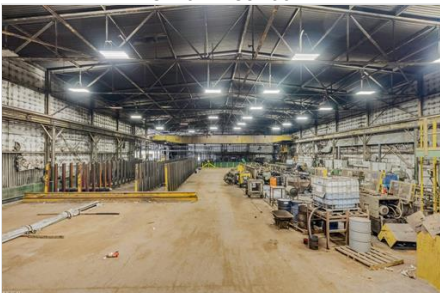
Miscellaneous room with concrete floors
