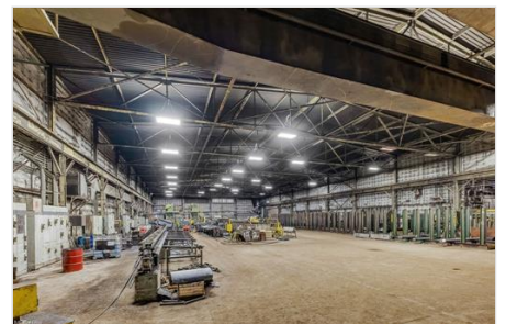
View of miscellaneous room
