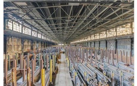
View of misc room
