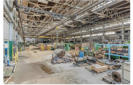
View of miscellaneous room
