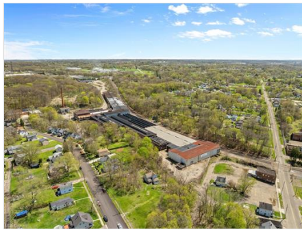
Drone / aerial view featuring a view of trees
