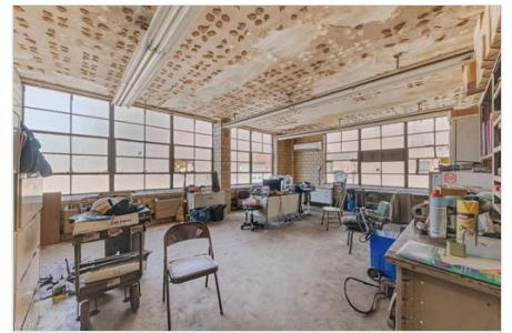
Miscellaneous room featuring a garage, unfinished concrete flooring, and a wall unit AC
