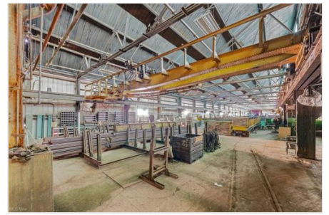
View of miscellaneous room
