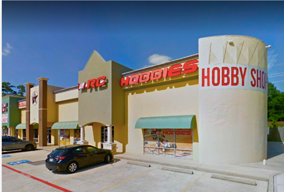
Front View (Awnings & Signage)
