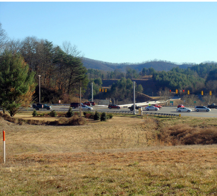
View of Underground Utilities - At right-of-way; surplus land available for parking lot.
