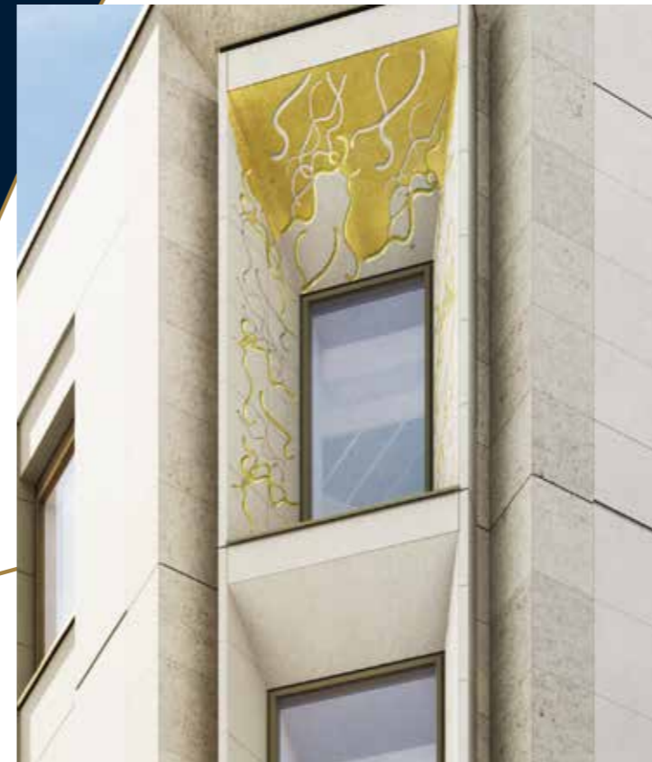
Finely detailed engraving, accentuated in gold, highlights the windows on the corner of Duke Street St James's and Jermyn Street.
