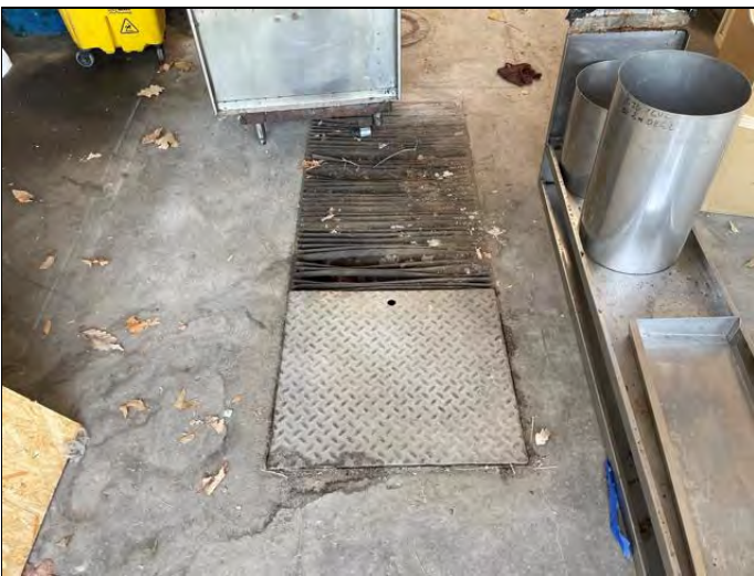
23. Interior – shop, oil pit
