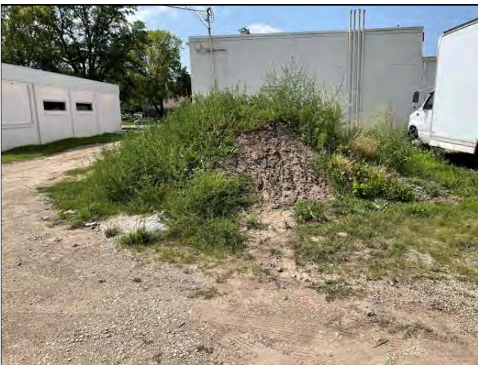
11. Soil debris pile
