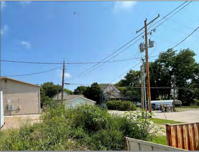
13. Pole-mounted transformer
