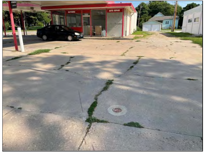
14. Typical monitoring well
