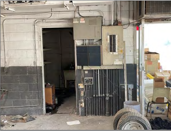
19. Interior – shop, mechanical room
