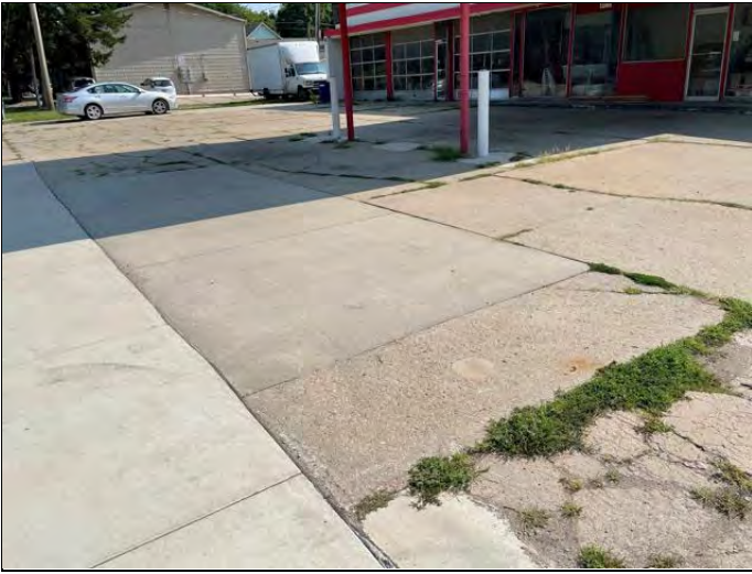
7. Reported former UST location
