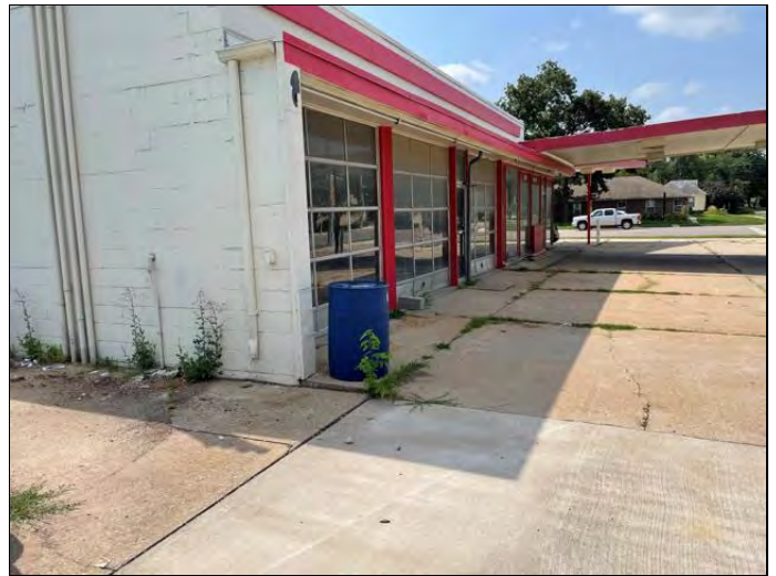
10. Oil storage drum
