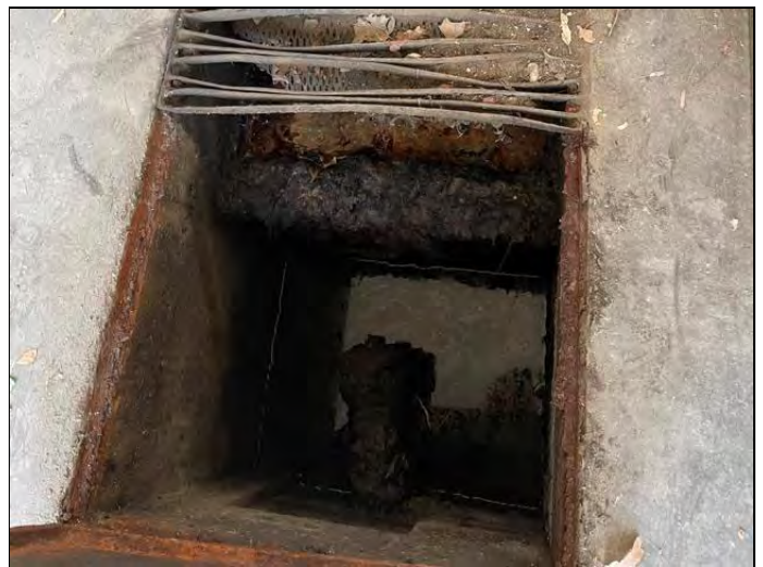
24. Interior – shop, oil pit
