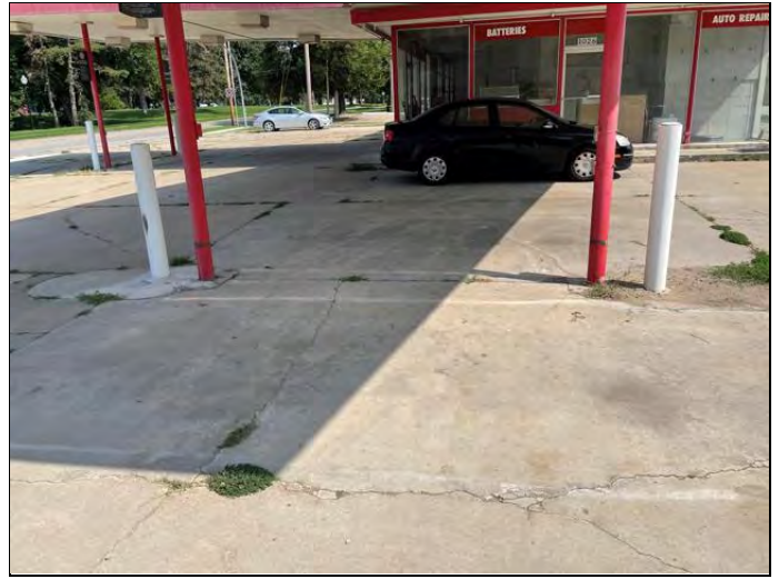
8. Reported former UST location
