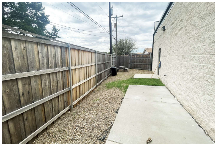
Back Yard Area
