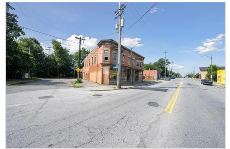
View of asphalt street with street lights, sidewalks, traffic signs, and curbs
