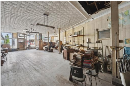
View of miscellaneous room Eastside
