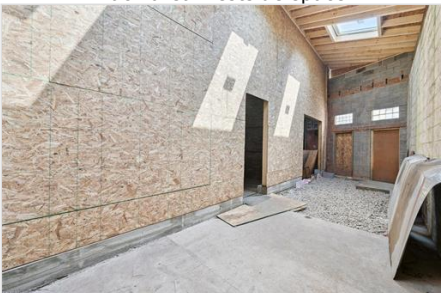
Misc room featuring a skylight
