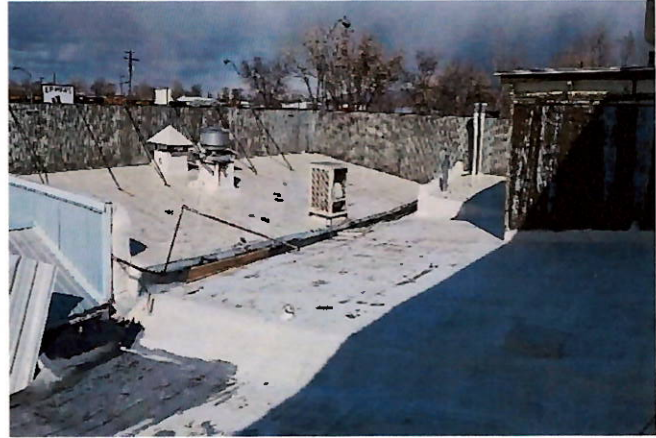
Picture 8 – Roofing with Mechanical
