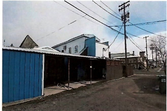
Picture 4 – Exterior Elevation (Looking North)
