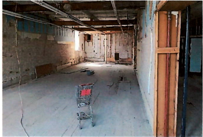
Picture 12 – Interior Framing
