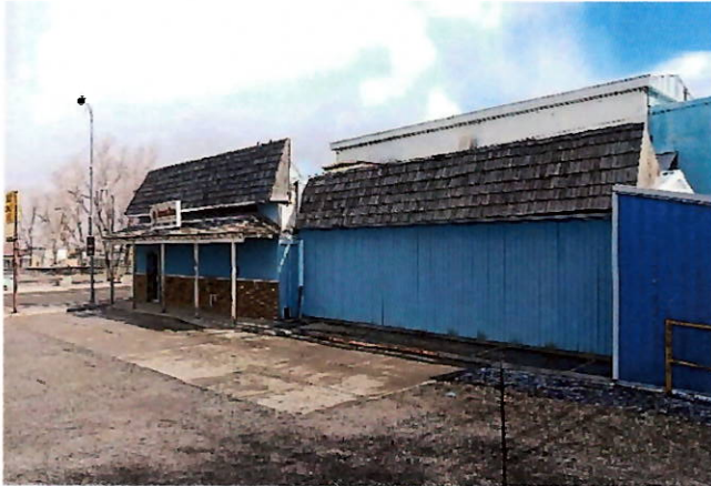
Picture 3 – Exterior Elevation (Looking East)
