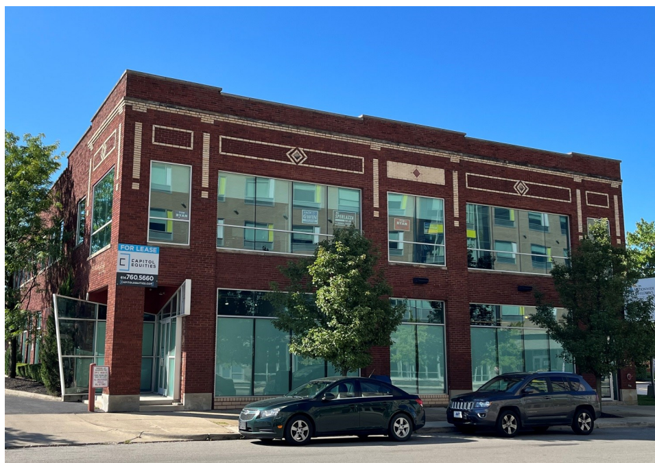
Dynamic Loft Office w/ 16' Ceilings
