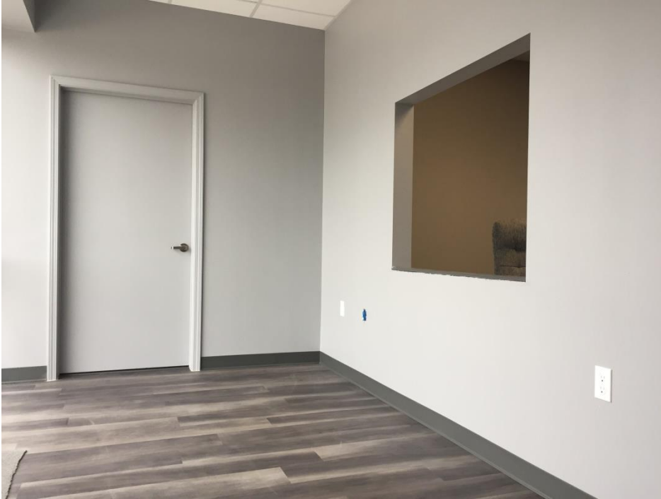
Finish-out of Building 6
