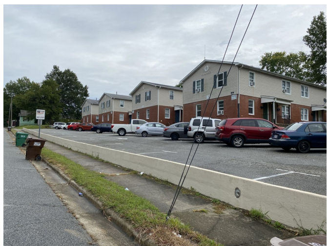
Representative two-story exterior and paved parking
