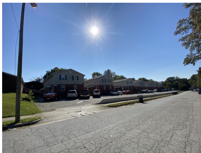
Representative single-story brick exterior
