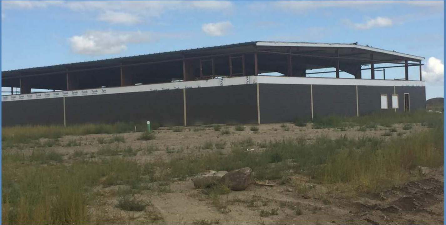
NEW GYMAGIC GYMNASTICS FACILITY UNDER CONSTRUCTION
