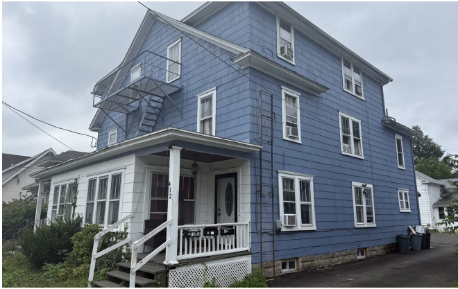
4-unit front building
