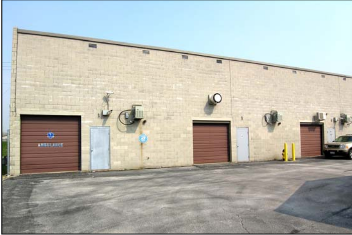
Rear of Building with Overhead Doors
