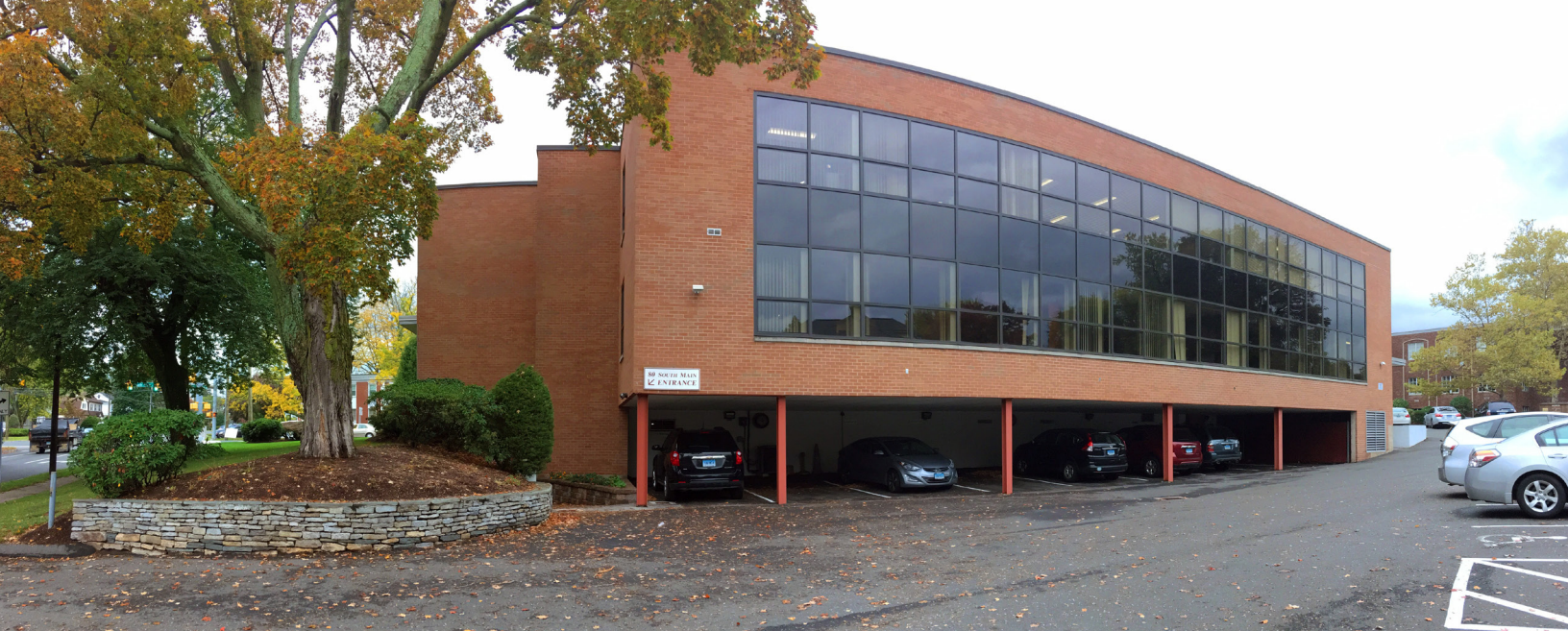
Under building parking
