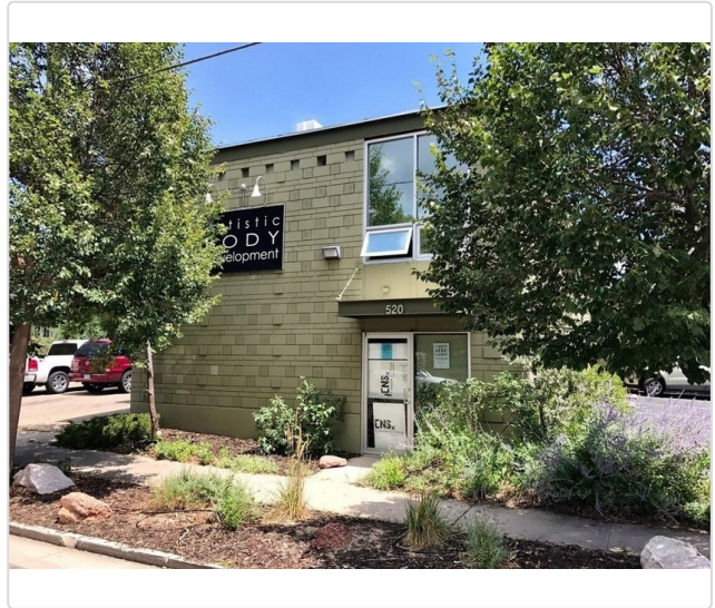
Building Exterior — 520 Cherokee St
