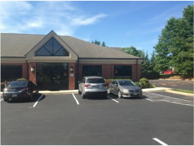
End unit of all brick professional building
