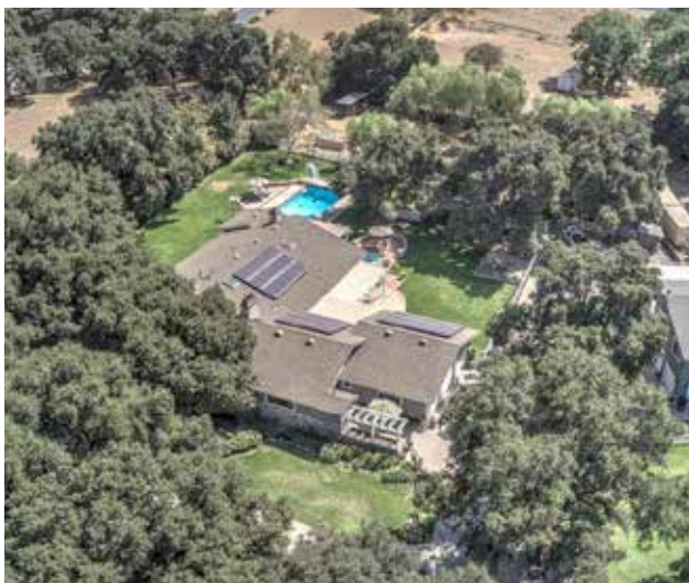
15323 IRON CANYON ROAD
