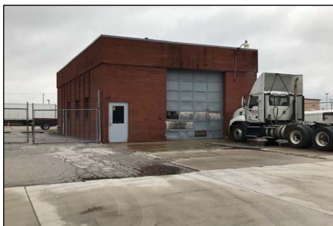
Drive in garage with 14' door
