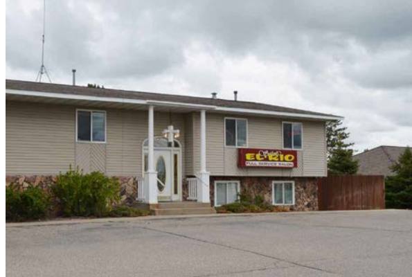
Front Entrance For Upper & Lower Levels
