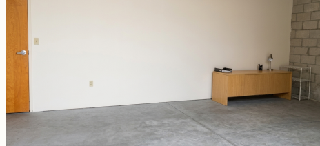
WAREHOUSE — WORK AREA
