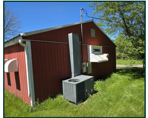
Building exterior — awning ventilation
