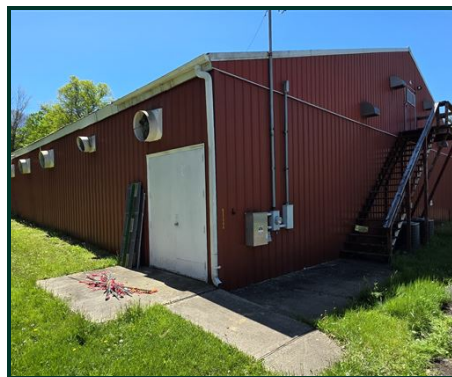
Utility building — drive-in access & apron
