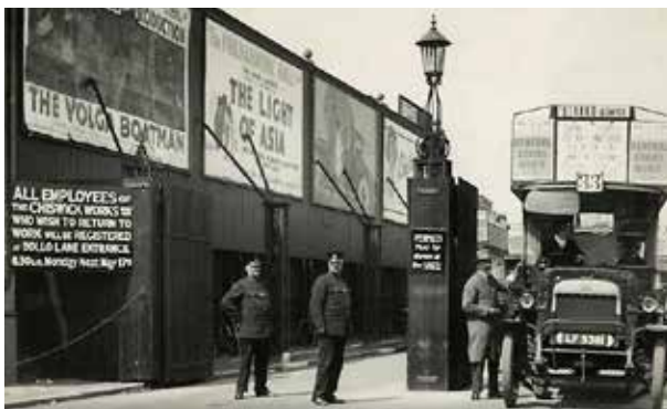
This photo (circa May 1926) shows the invitation to return to work posted at the Chiswick bus depot at the end of the General Strike (now the site of Chiswick Park).
