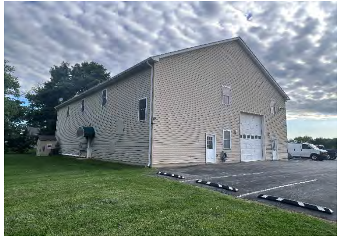
Rear View of Building High Bay Drive-In Door
