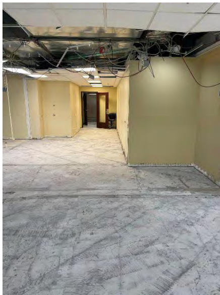
Open Area to Entrance
