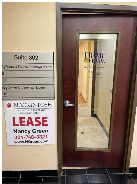
Exit Door from Suite To Common Hallway
