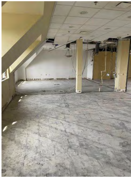
Interior View North
