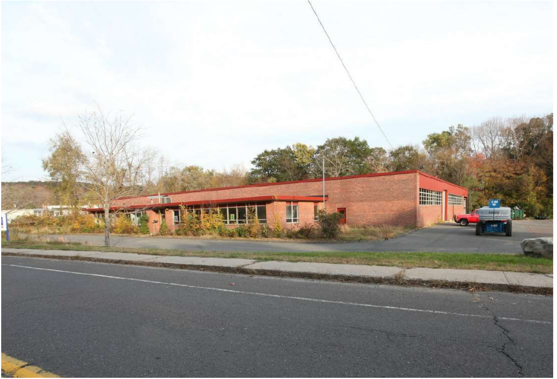
11 Skinner Street, East Hampton, CT - Subject Property – Exterior Photos – Front of Building
