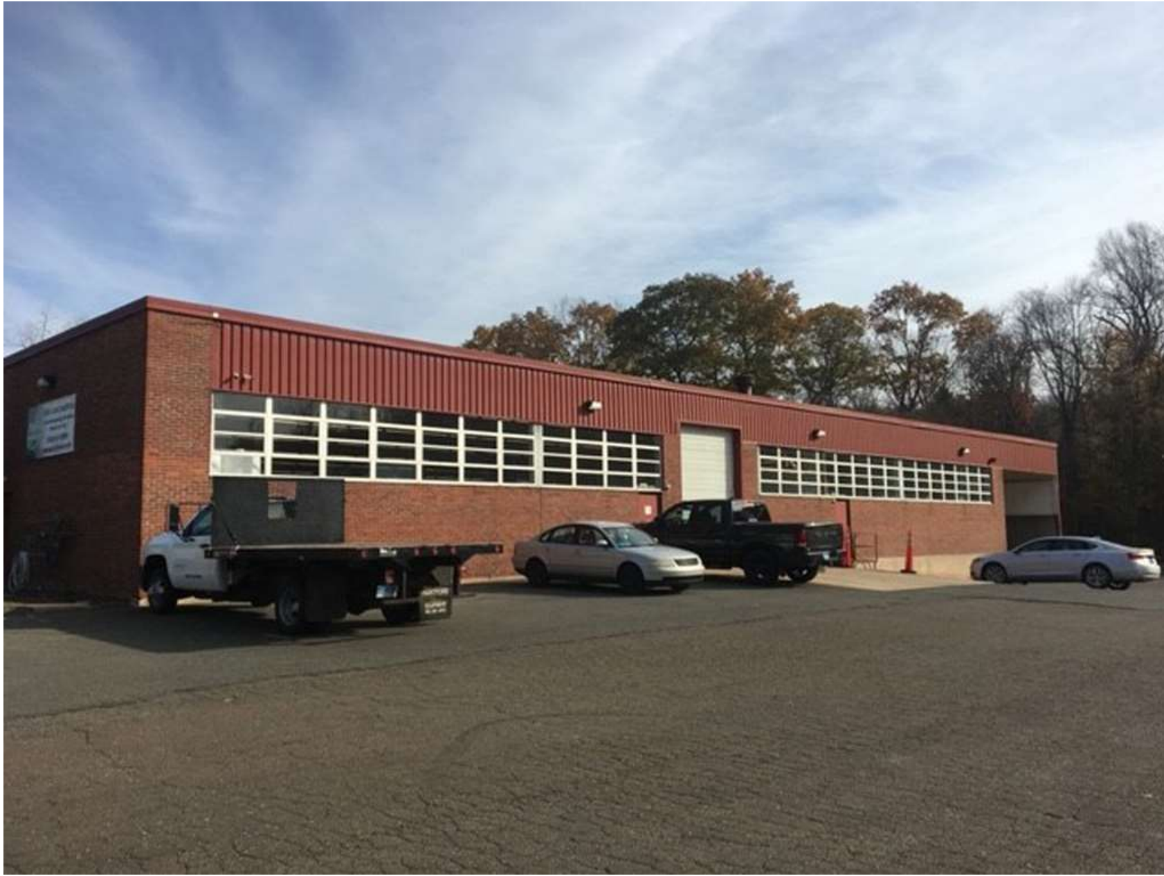
11 Skinner Street, East Hampton, CT - Subject Property – Exterior Photos – View of West Side of Building
