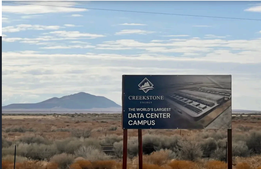
The gigasite being built in Utah by Creekstone is thought to be the world's largest data center campus. Credit: Creekstone Energy
