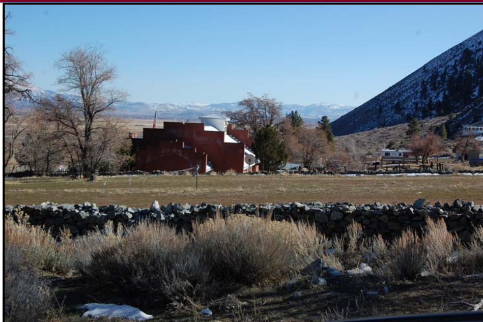
View from Northwest, US Post Office in background
