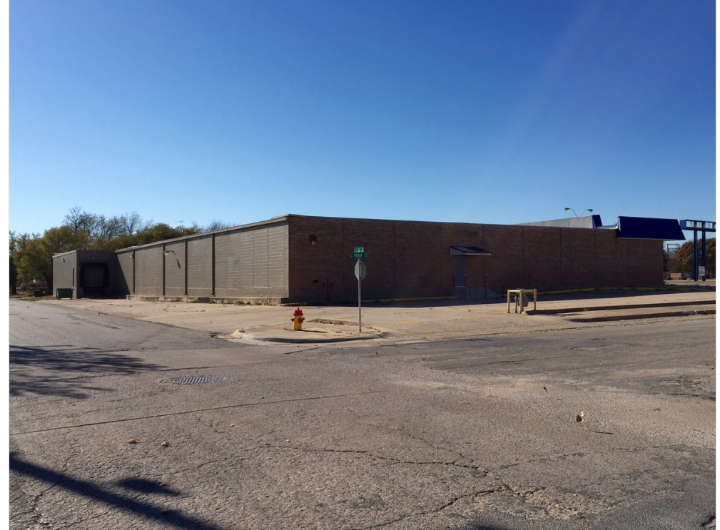
Full Loading Dock with easy access
