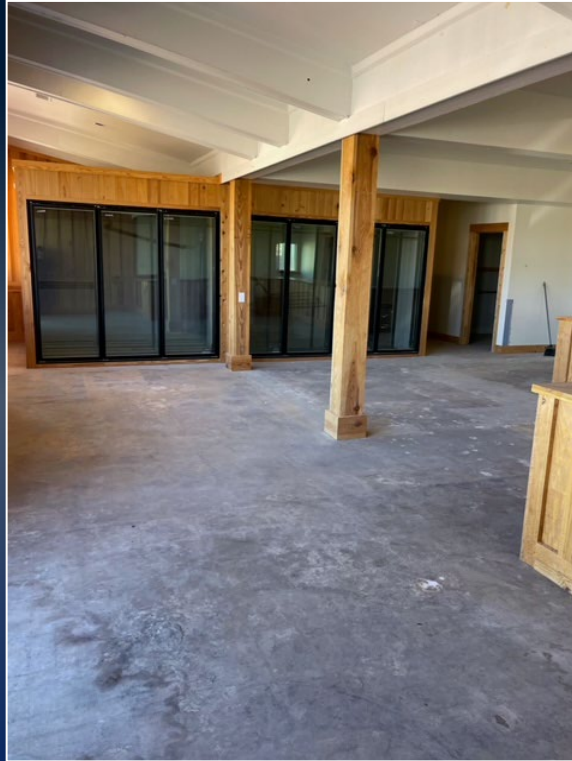
Building 1 – Walk-in Cooler
