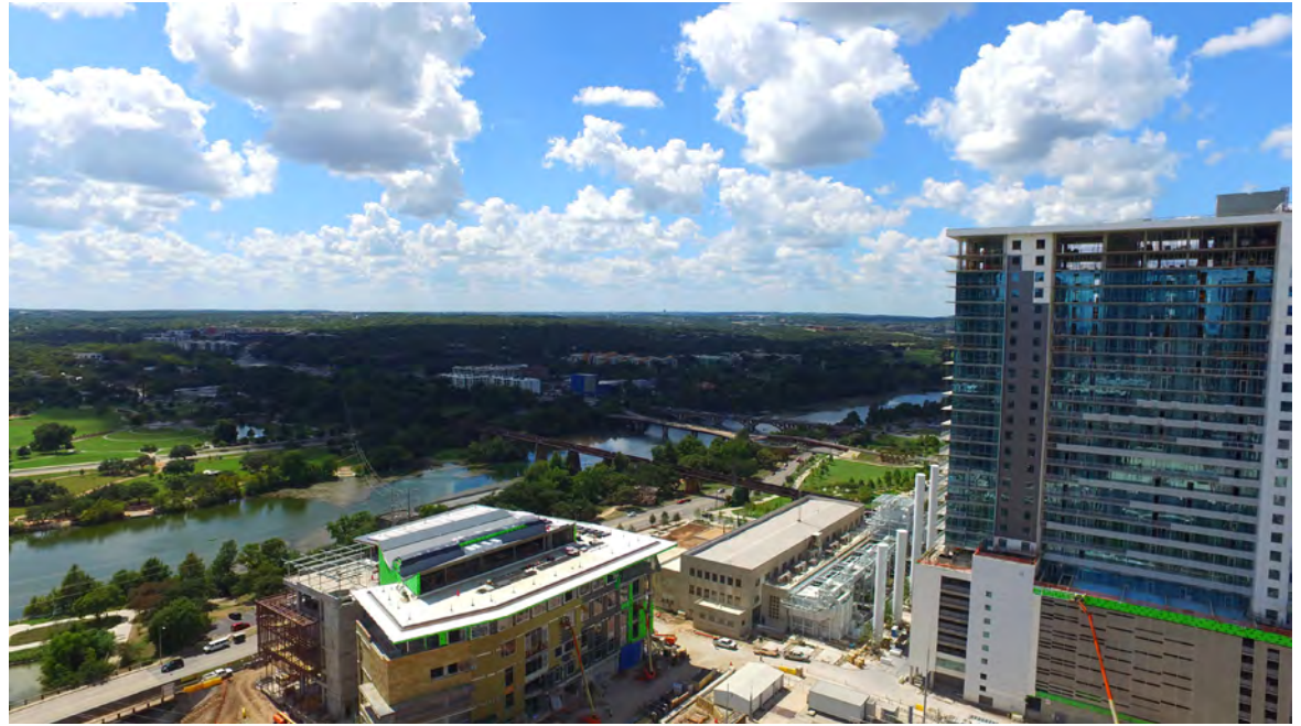
Floor 21 Looking South
