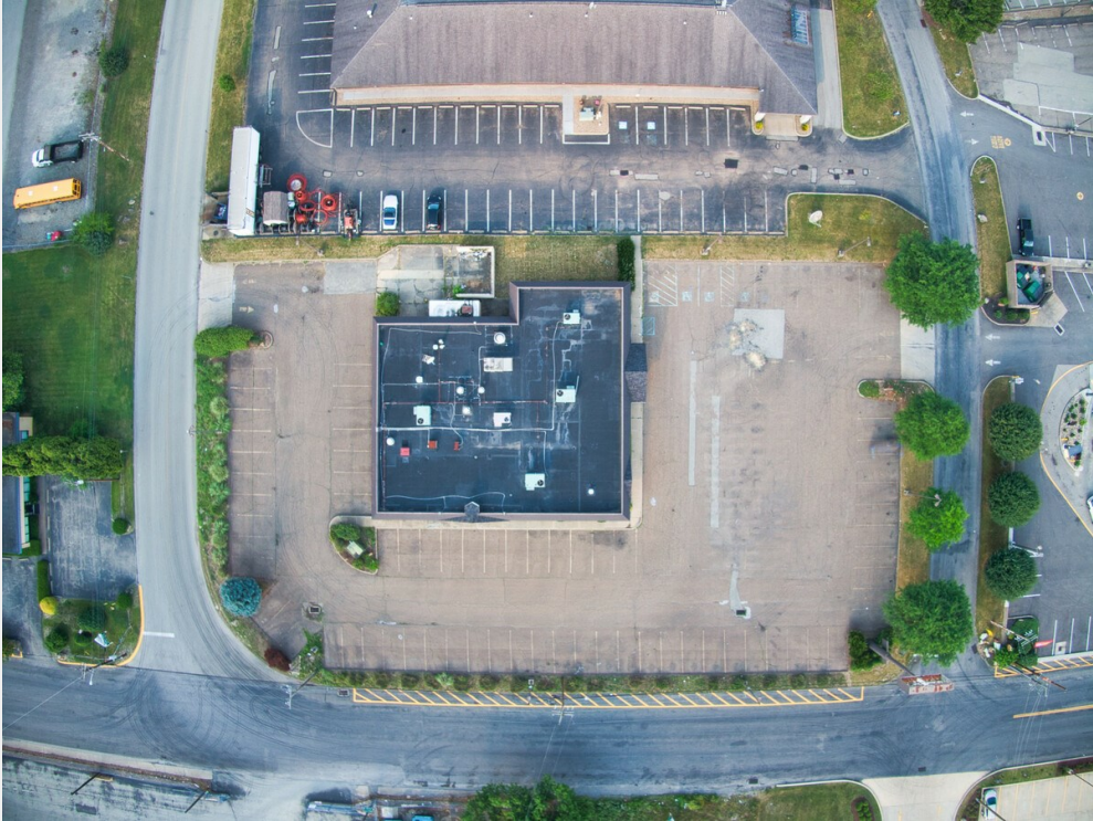
Aerial View of Lot
