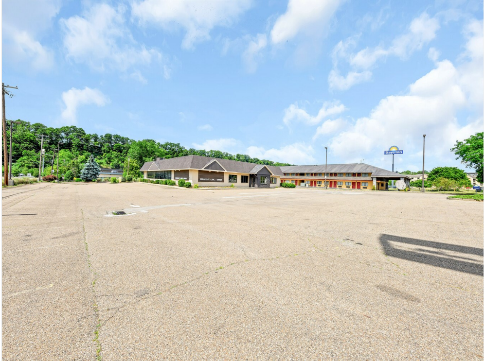
Angled ground level view of lot
