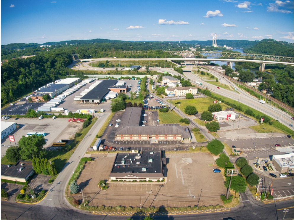
Ariel view of Pennsylvania Turnpike Interchange
