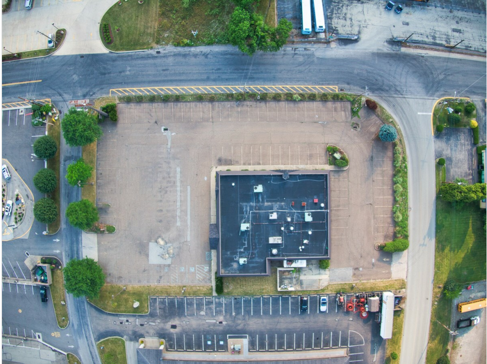
Aerial View of Lot
