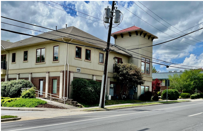
ADA-Compliant Rear Ramp & Corner Elevation
