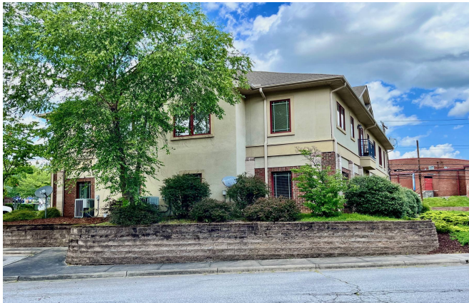
Rear Elevation — Mature Landscaping & Retaining Wall
