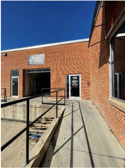
View of Dock Door
