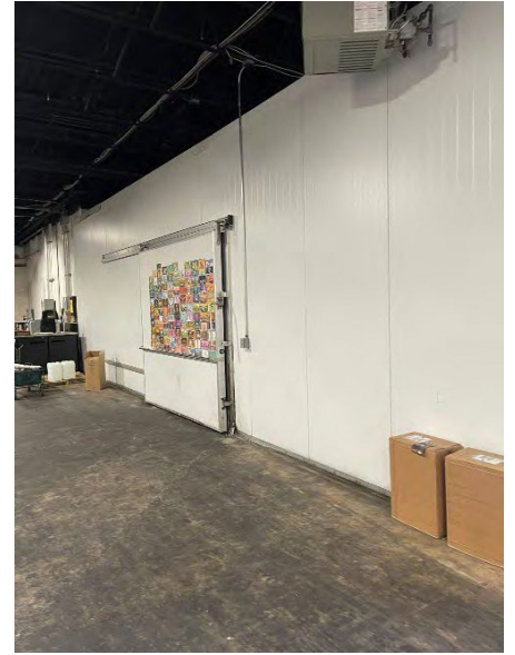
Inside View of Cooler Room
